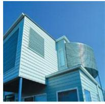
Hardboard products must be fixed using special fasteners that allow flexibility and board movement due to ambient moisture variations.
